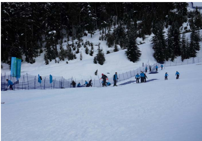
Installing one type of B safety systems, usually in triple layers
